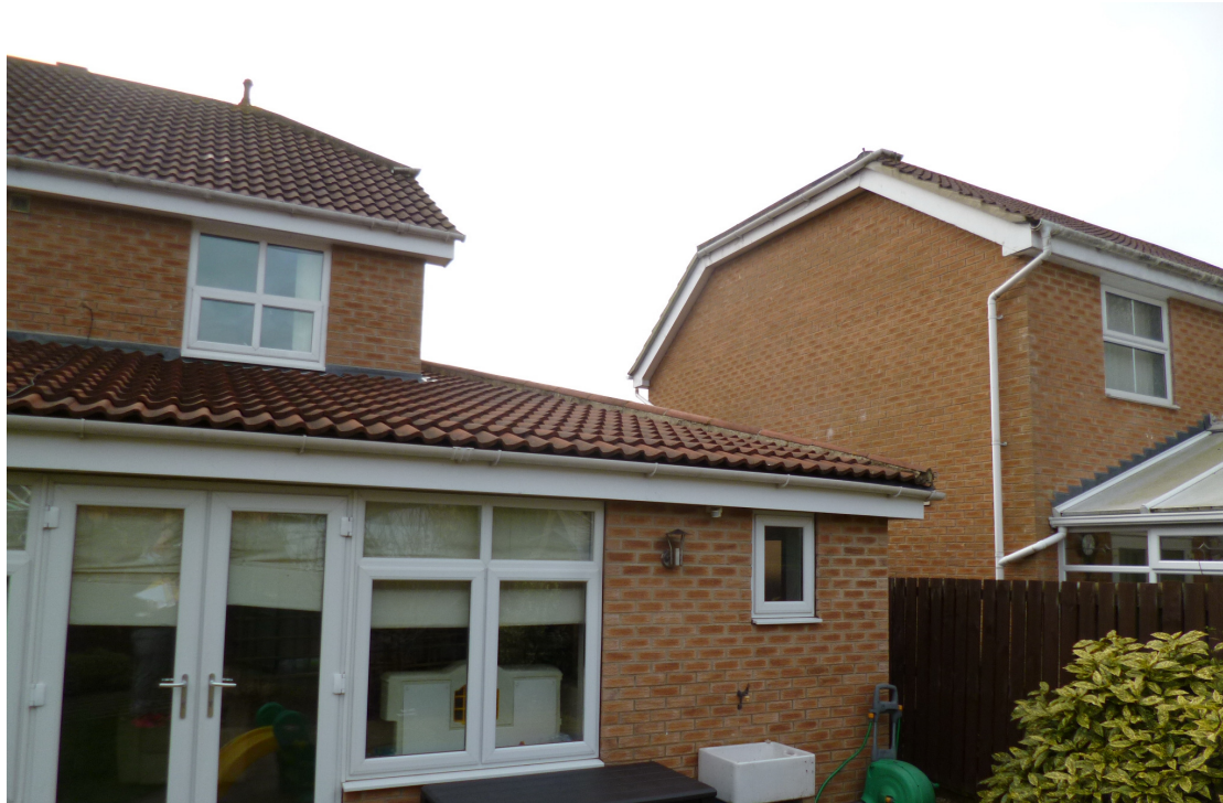
View to side/rear of No 44
